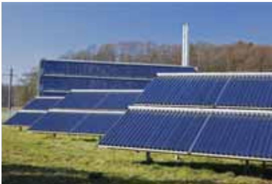
Figure 3: Vacuum tube collectors in Büsingen, Germany
