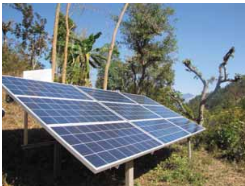
Fig. 7: Solar water pumping array (9s x 1p) rated at 1.26 kWp used for irrigation by the Taule village farmers.
