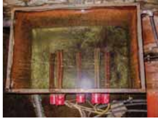
Fig. 3: Resistive water heater elements are used to dissipate energy into the turbine's exhaust water.
