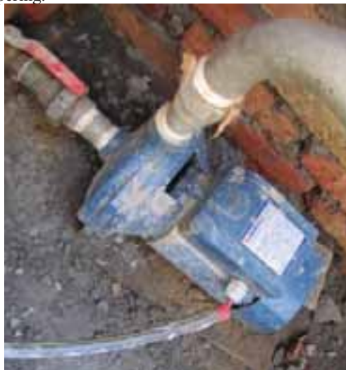
Fig. 2: Pedrollo (Italian) surface centrifugal AC solar pump used in Odaltal village of Surkhet District for rice irrigation.
