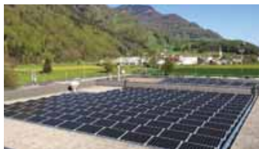
Figure 10: P&D project Lintharena in Näfels (CH). Uncovered PVT collectors for the pre-heating of groundwater providing heat to a heat pump (Rohrer, 2016).
