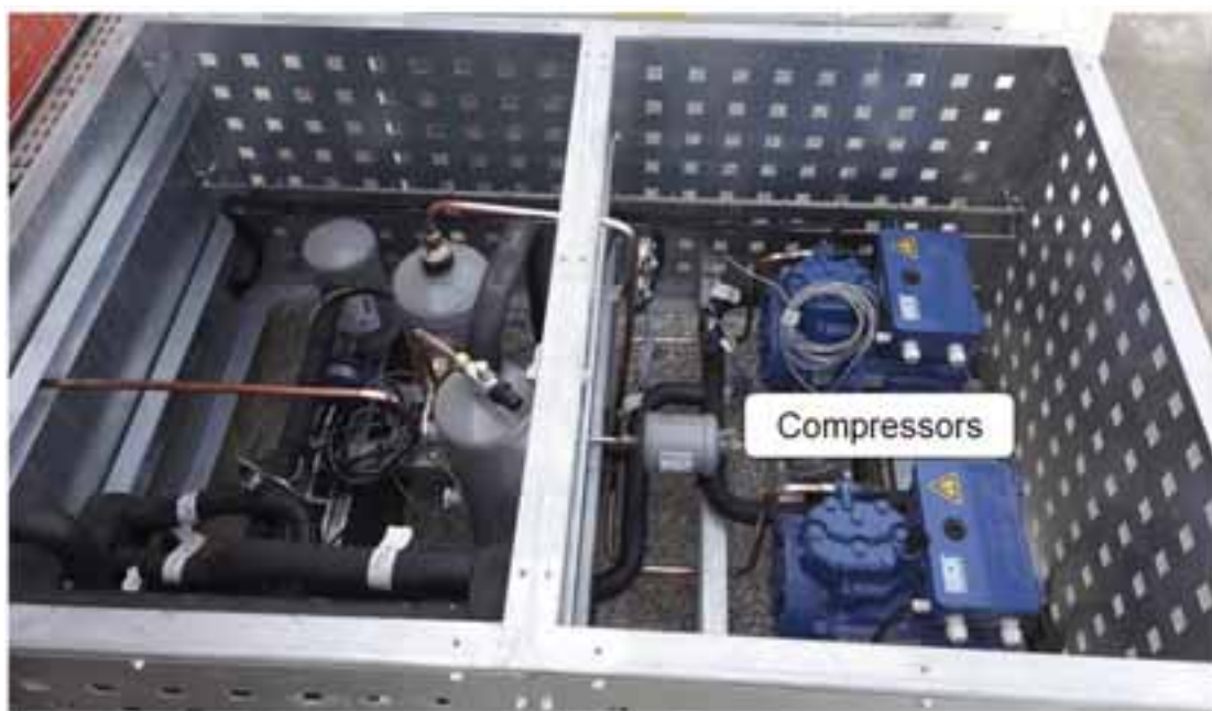
Fig. 5: Picture of the Two parallel-mounted semi-hermetically compressors
