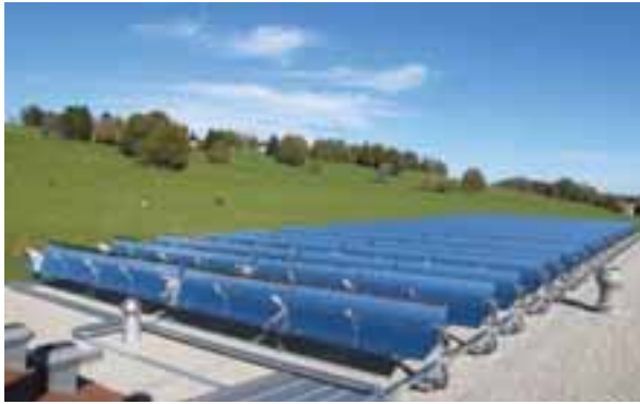
Fig. 1: SPHP in Saignelégier, 1000 m above sea level, 627 m 2 (aperture) PTC collectors with axis orientation NS with 18° deviation counterclockwise
