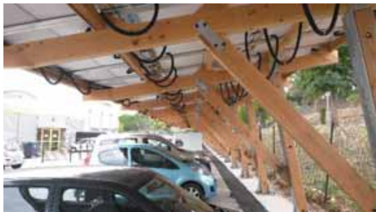
Fig. 3: picture of the PV/T canopy for the municipal swimming pool of Perpignan (France)
