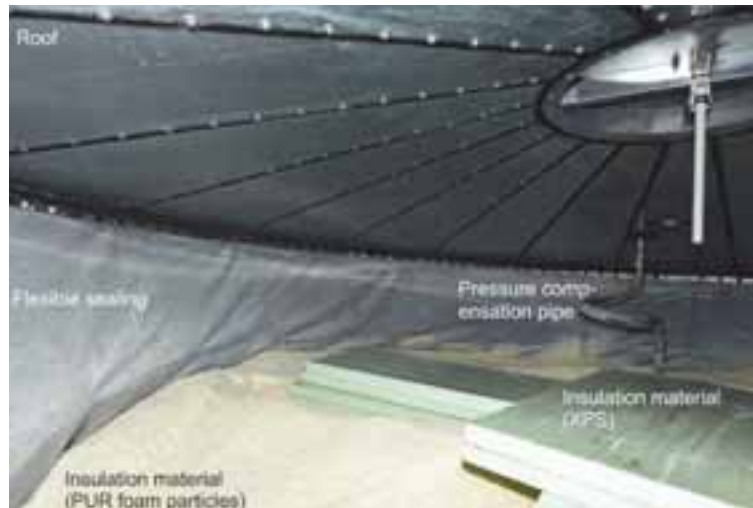
Figure 8: Laying of XPS panels on the PUR foam of the floating ceiling in the attic during the construction, July 2017
