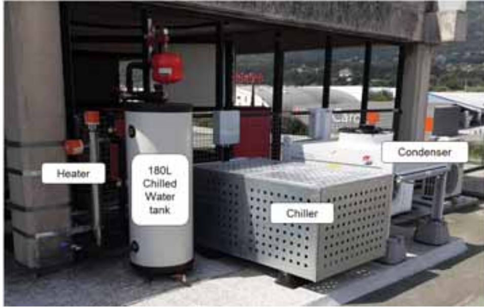
Fig. 6: Picture of the global chiller installation installed on the Atisys top roof
