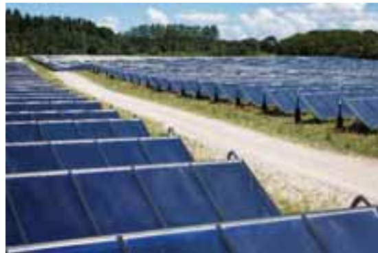
Figure 4: High-temperature flat plate collectors in Dronninglund, Denmark
