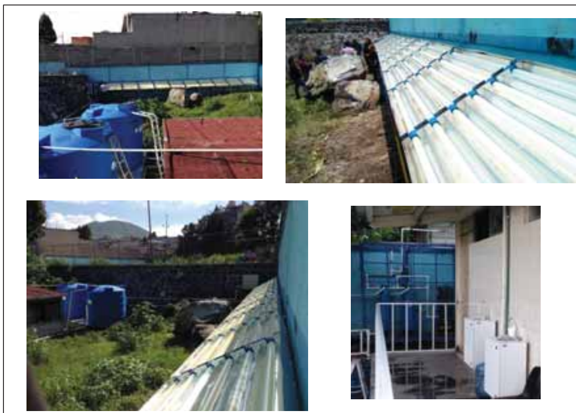
Fig. 14: Photochemical treatment system coupled to potable water train system and drinking water dispensers
