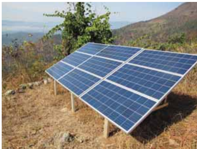
Figure 10: Solar power array using German made Komaes140 Wp PV modules (9s x 1p) for t Pokharikada using a Grundfos submersible centrifugal solar water pump.
