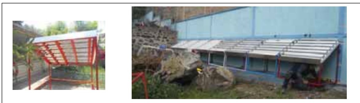
Fig. 11: Parts joint and aliening-fastening on the wall
