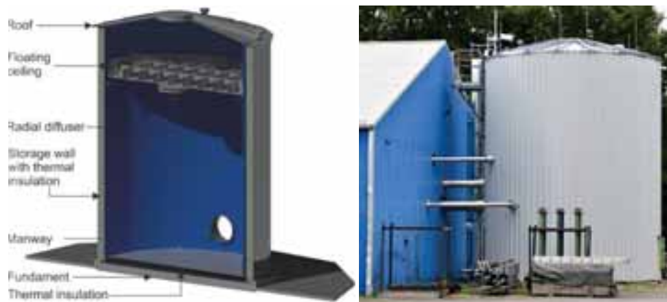
Figure 9: CAD-Visualization (left), panelling with trapezoidal sheet metal (right), July 2017
