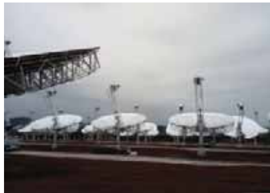
Fig. 10: Dish Stryn solar thermal power system in Tongchuan
