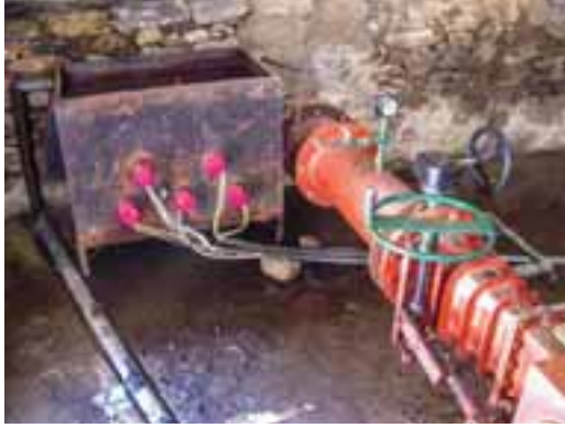
Fig. 2: Traditional water heater “dumb” dump load in MHP (micro-hydro-power) plant in Nepal
