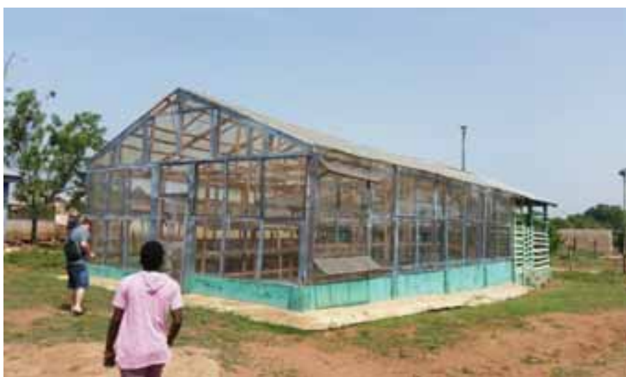
Fig. 1. 5tonne capacity dryer located in Ejura
