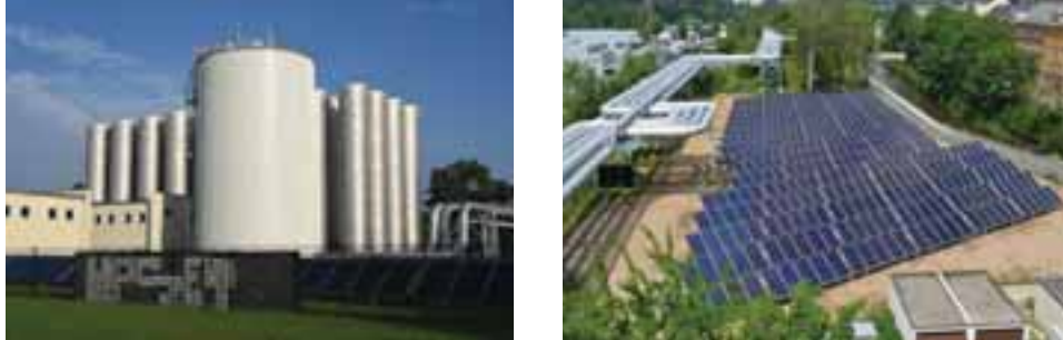
Fig. 3: South solar collector field and two-zone storage (left) and north collector field (right) in the Brühl system, Chemnitz.
