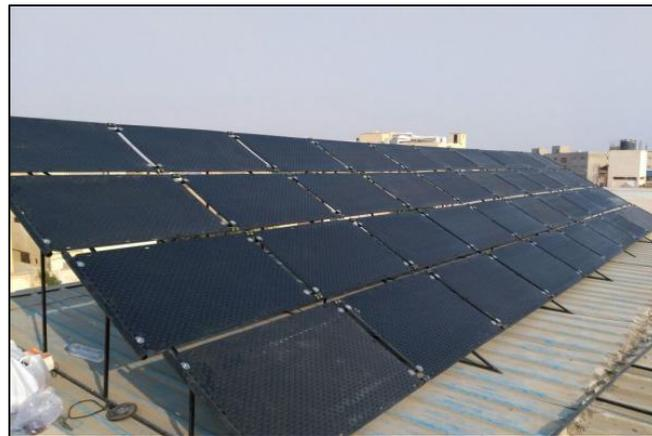
**Fig. 2 Example of PVs Arrangement on Roof Tops  $\beta = 30^\circ$  (tech waves, 2019)**
